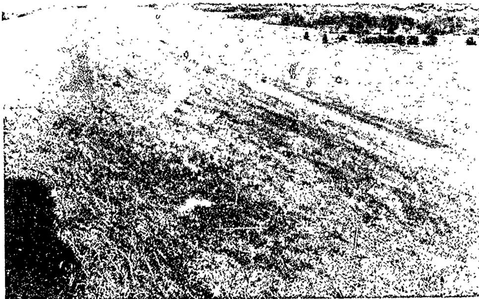
PHOTO 2. View of the grass covered D/S slopes of dam. Note the flat berm in the background over the old slide area, Sep 83
