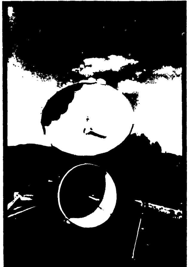
Fig. 1. 6.1 meter antenna used as a hub (shown in background) and 1.8 meter VSAT (shown in foreground).
