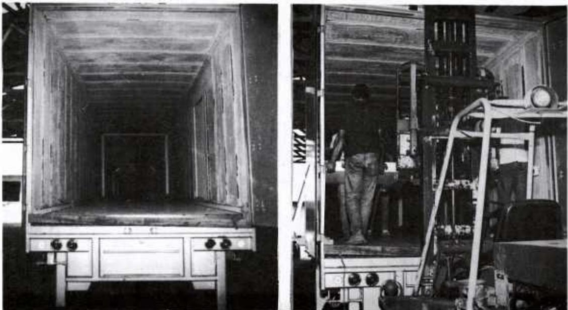
Figure 2. Views of MFL interior showing trailer side post construction after spraying with acoustic gapping material (left) and the 4-in thick acoustic panels in the process of being installed (right).
