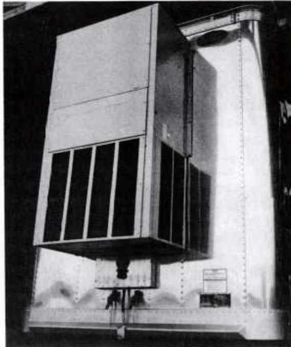
Figure 10. View of heating and air conditioning unit installed on the front vertical surface of each MFL. The unit is isolated from the trailer frame by neoprene gaskets to minimize the transmission of acoustic and vibration noises to the MFL superstructure.
