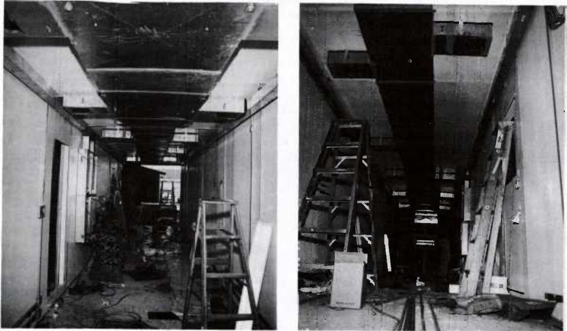
Figure 3. Interior of MFL after installation of the 4-in thick floor, sidewall, and ceiling acoustic panels but prior to installing the 3-in thick dropped ceiling panel.
