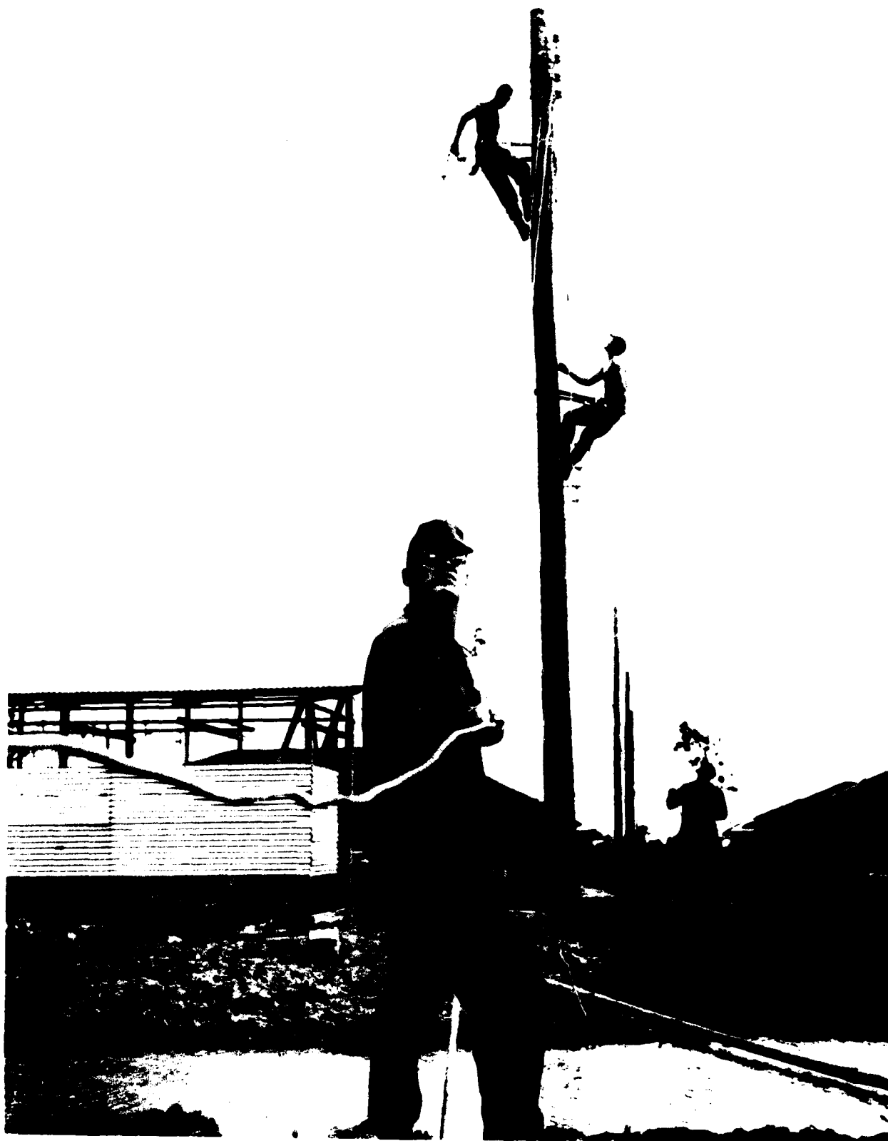
Members of Company C, 9th Signal Battalion, install power cables for the THAI "Queen's Cobra" Regiment, at Camp Martin Cox, Vietnam, 1967.
