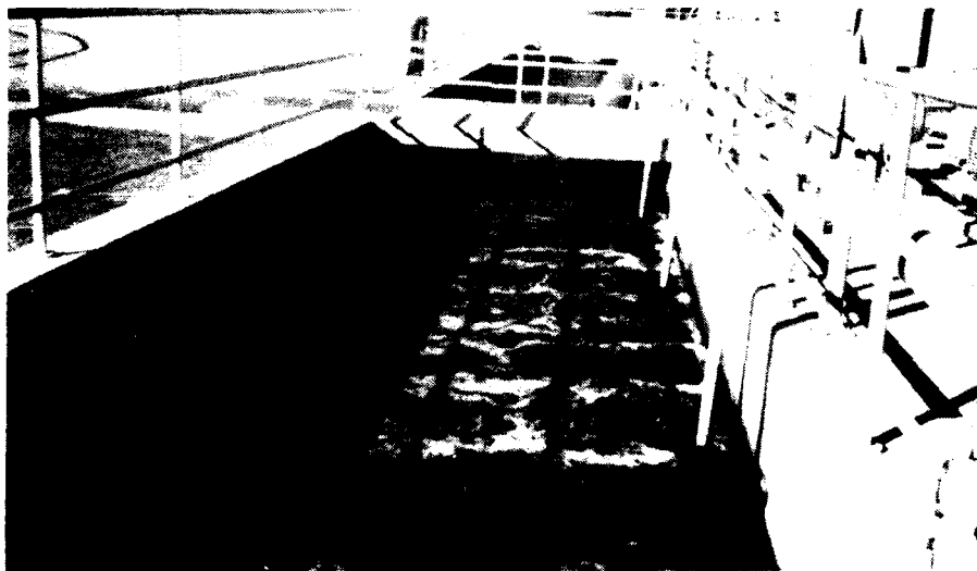
Figure A4. Aerated solids contact tank at Tolleson wastewater treatment plant. The blowers for the solids contact tank are above ground at this location.
