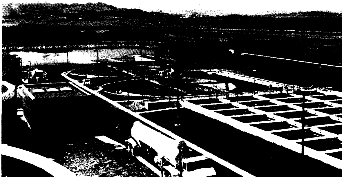
Figure A1. Overview of the Elk River trickling filter/solids contact treatment plant at Eureka, CA. Primary sedimentation tanks are in the right foreground. The L-shaped aerated solids contact tank can be seen between the primary and secondary clarifiers. Secondary clarifiers are in the center, and the effluent holding pond is behind the clarifiers. (Source: Brown and Caldwell Consulting Engineers. Used with permission.)
