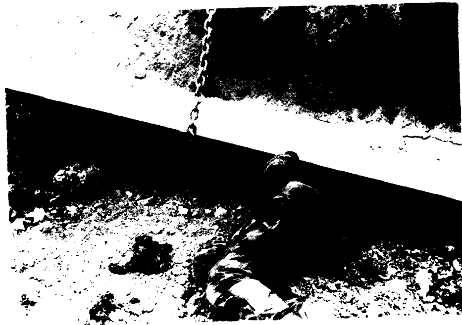
Figure 36. An operator crawling beneath the dozer blade in order to attach the chain to a shackle.
