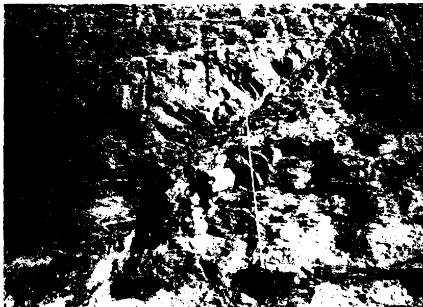
16. Fault at one on one slope, in impervious core zone, 23+56S, 0+12D.
