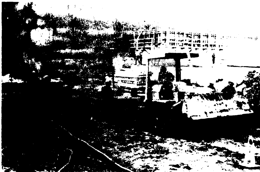
2. Sawing shale for lower crossover trench at 7+39D. Monolith R-29 in background.
