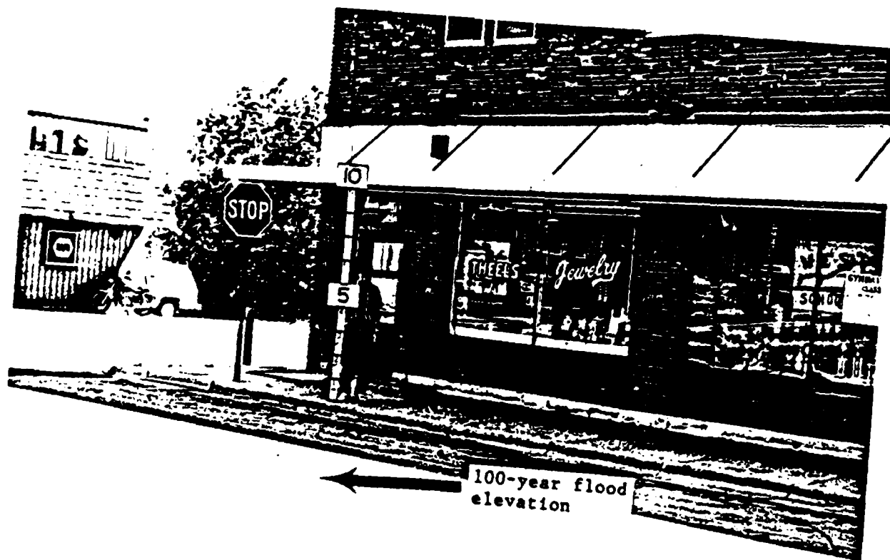
Site 5 Front, August 85, Watertown, MN PHOTOGRAPH 2
