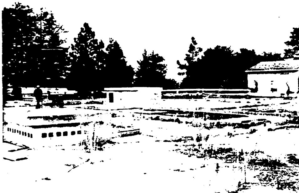
Lower launch site at Barley Flat. Note the concrete block structures added when the silos were converted to civil defense facilities following closure of the Nike base.
