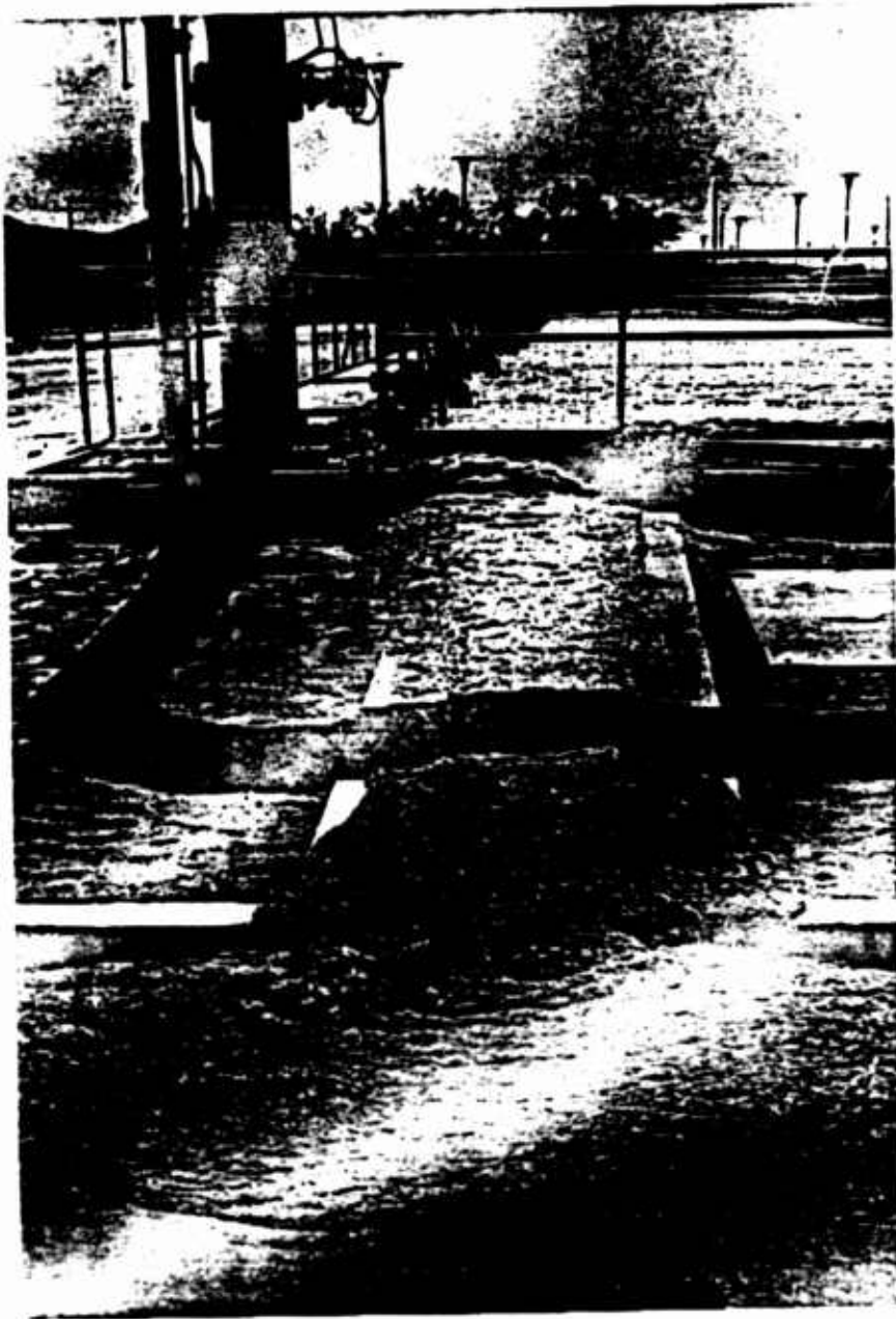
Figure 1: Severe Foaming at WWRRA Treatment Plant
