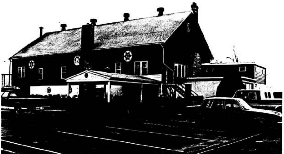
Illustration 3 View of the Officers' Club (Building 79). This wood-frame structure set on a stone foundation was originally constructed around the turn of the century as a barn. It was remodeled and converted into the Officers' Club in 1942. (Source: Field inventory photograph, 1984, Barbara Hightower, Building Technology, Inc.)
