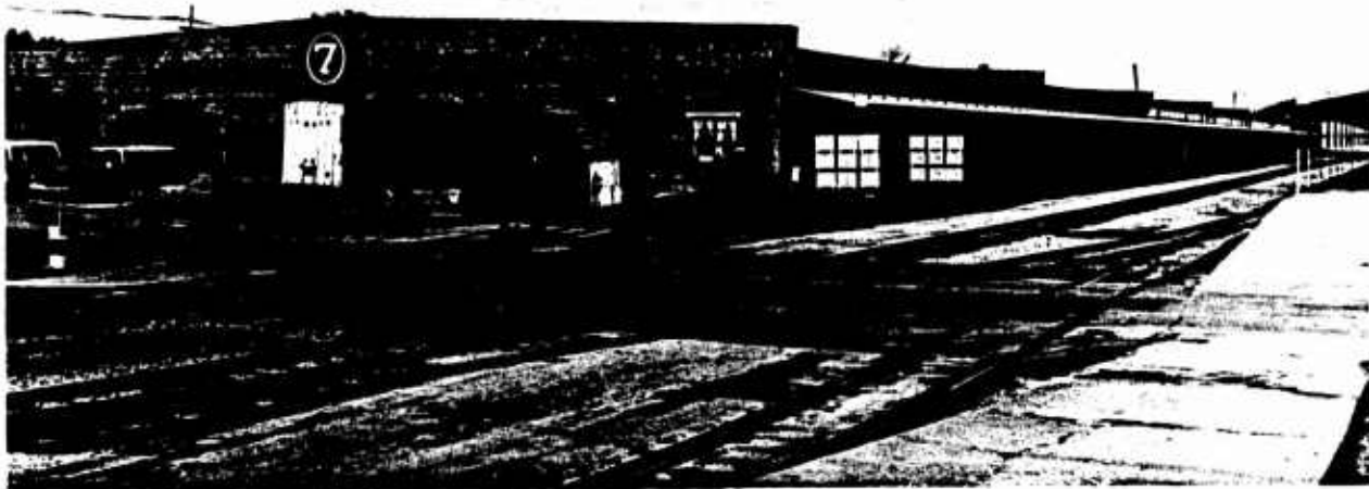
Illustration 4 View of Building 7. This brick and clay tile structure was one of eight warehouses built during the depot's initial phase of construction in 1918. (Source: Field inventory photograph, 1984, Barbara Hightower, Building Technology, Inc.)
