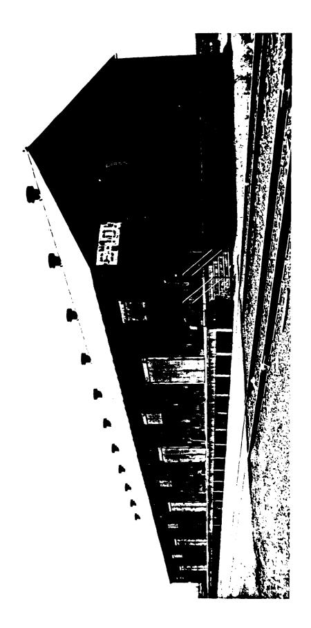
Building 26. This hollow clay tile structure is one of 11 standard above-ground magazines erected in the ammunition storage area in 1942. (Source: Field inventory photograph, Christy Johnson McAvoy, McIvyn Green & Associates, 1983) Illustration 3
