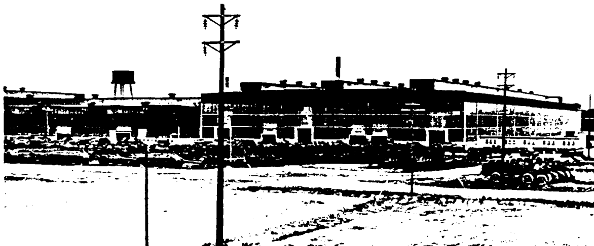
Illustration 3 Historic photo of Building 147, probably taken shortly after World War II. In particular, note the original glazing. (Source: General Dynamics)
