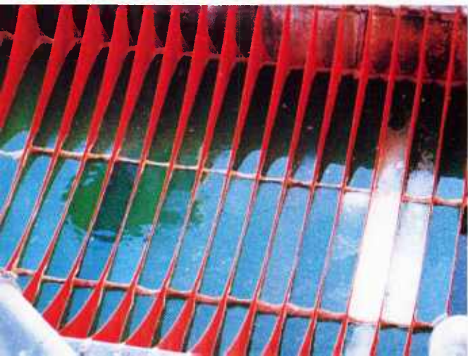
Above, Shuttle 51-L on Kennedy Space Center Pad 39B in the early morning of launch day. Temperatures were well below freezing, as indicated by the lower left photo, which shows thick ice in a water trough despite use of an anti-freeze solution.
