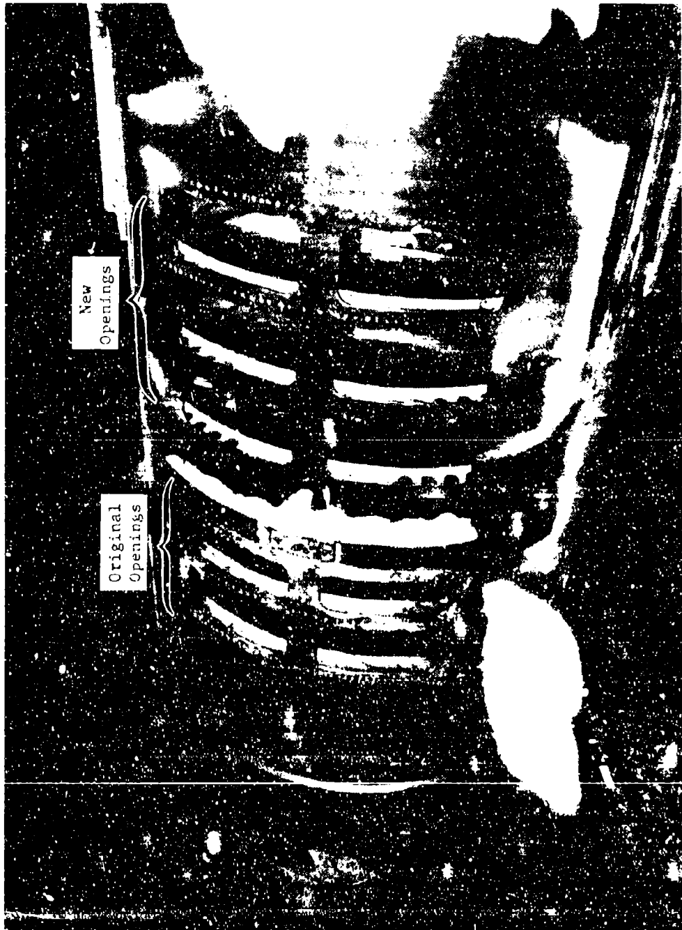
Photo 8. Water Tank Jettison Door Openings
