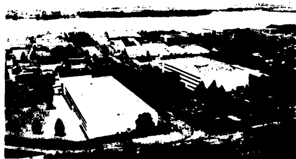
A unique combination of a current photograph and an artist's concept of how NRL could look in the year 2000. Under the CFIP, certain buildings will be renovated and modernized while other temporary buildings will be torn down to make way for new construction.
