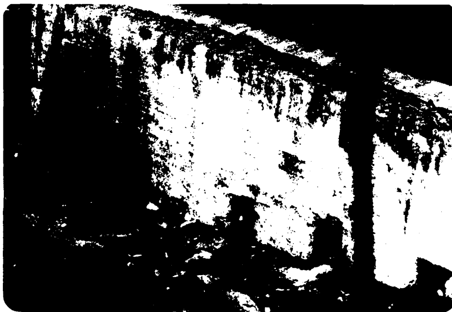
6. View from left side downstream showing typical deterioration of spillway face, old sluiceway (larger opening), and pressure relief drains (smaller openings)
