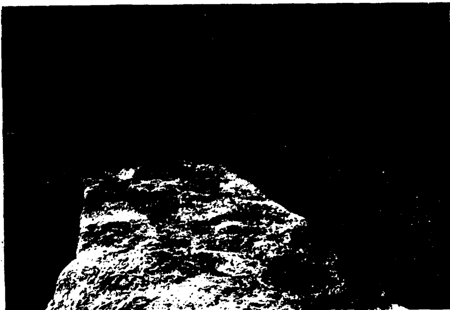
17. ERODED DOWNSTREAM FACE OF WORONORO (60 FOOT) DAM. NOTE DETERIORATION AT JOINTS AND CRACKS.
