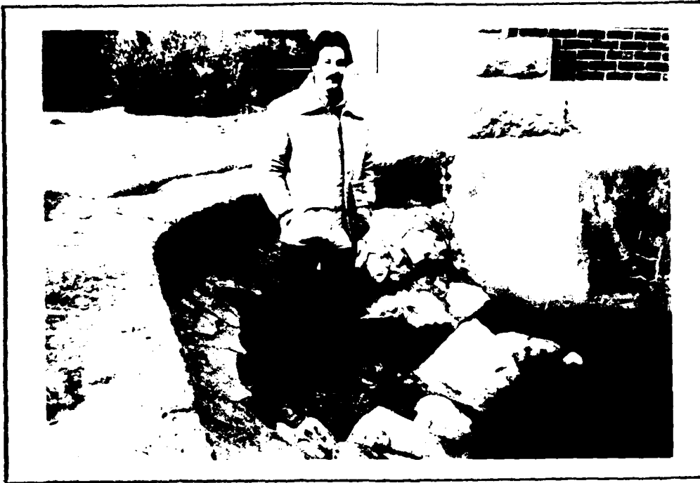
3. DISPLACED ROCK RIPRAP ON THE UPSTREAM FACE OF THE DAM NEAR THE GATEHOUSE. (10/17/79)
