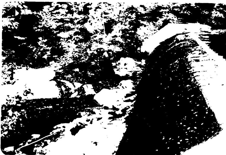
2. View of right abutment from left side of spillway showing bedrock outcrops at abutment and under spillway
