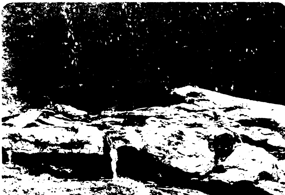
9. Detail of deteriorated concrete on downstream side of spillway
