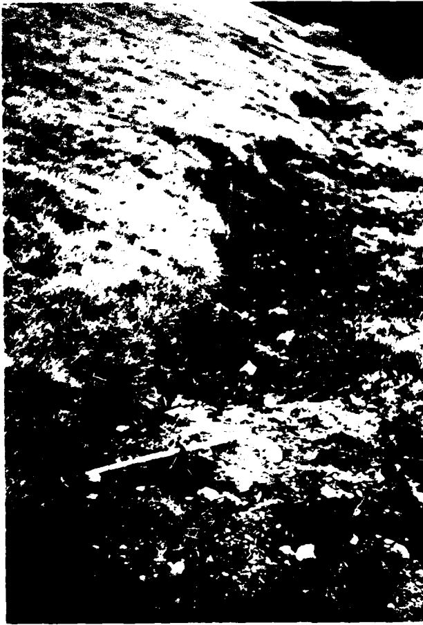
6. RULE EXTENDING 4.5 FEET INTO HOLE AT TOE OF DAM. SEE PHOTO 5 FOR LOCATION OF ERODED AREA.
