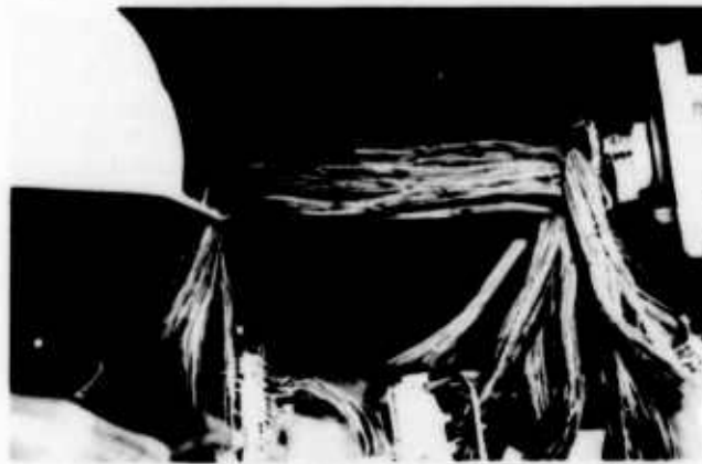
FIG. 5 CABLE SPLICE IN PROGRESS
