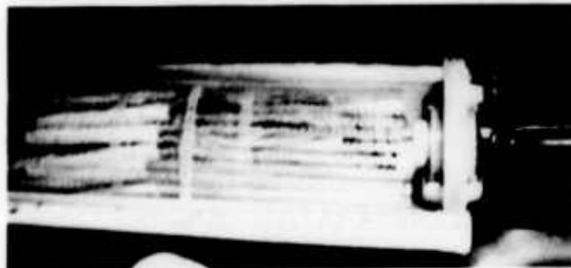
FIG. 6 COMPLETED SPLICE
