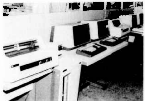
Photo 2 Computer room after installation
