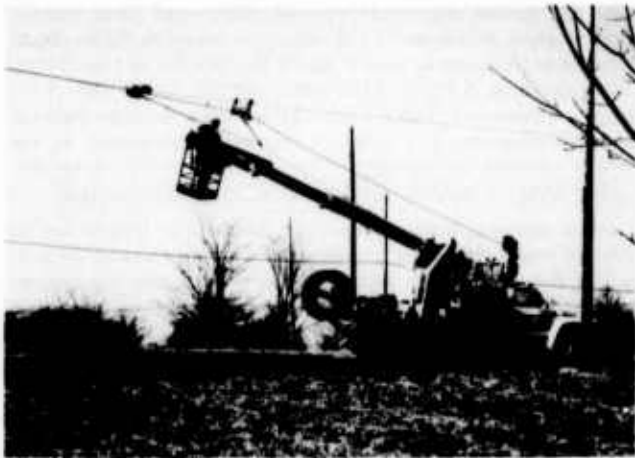
Figure 1. Line Truck Placing Aerial Lightguide Cable.
