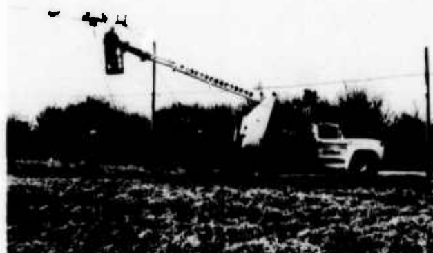
Figure 10. Use of Running-Line Dynamometer to Measure Low Cable Tension.
