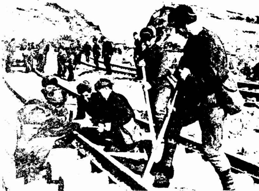
Building a railroad. Central Front.
