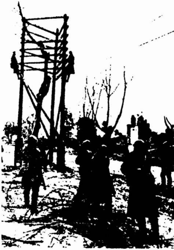
Restoring communication lines.
