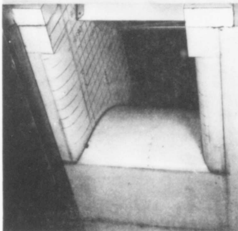
Upstream face of spillway bay without bridge.
