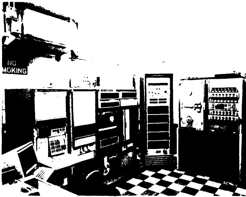
Fig. 7 - Computer Control System
