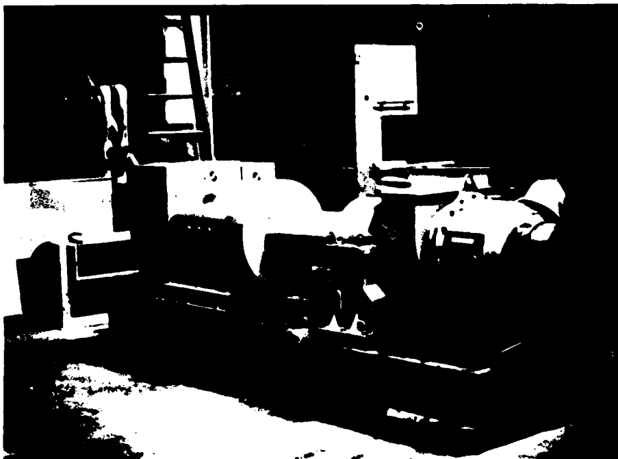
Figure 8 — Gas Turbine on Isolated Floor
