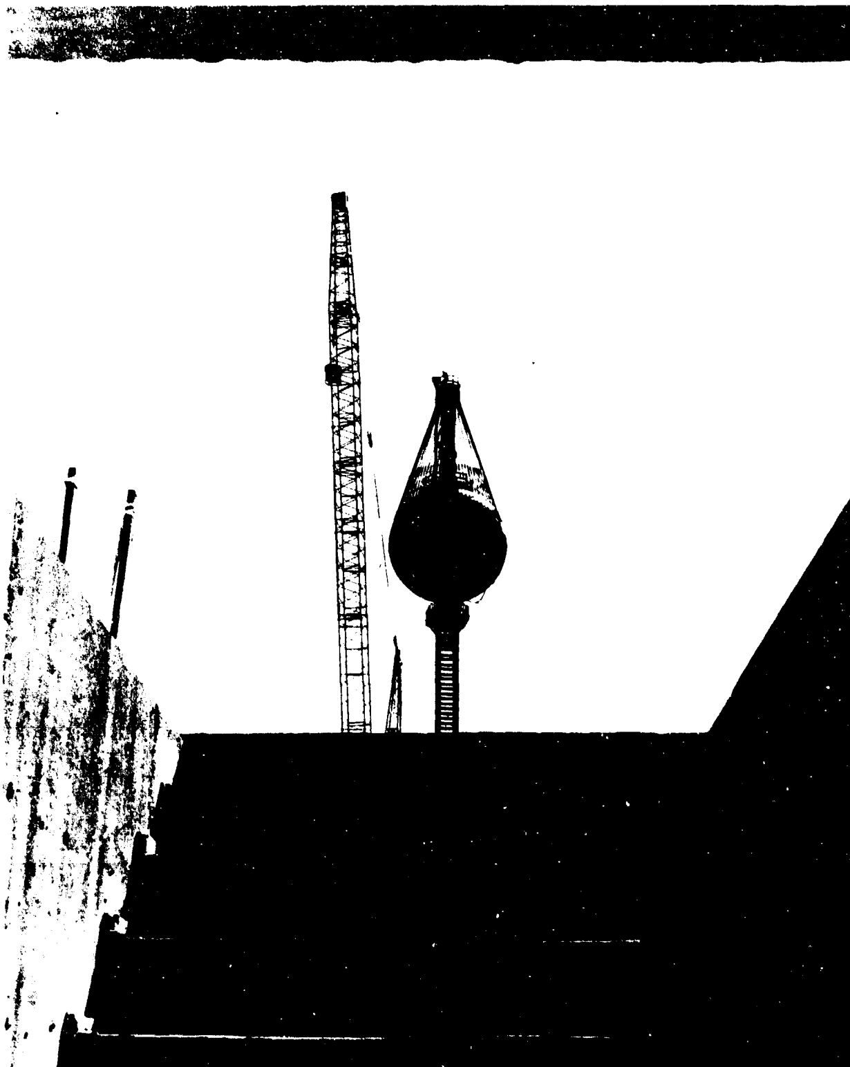
Figure 2.3. Charge tower as seen from entryway interior.
