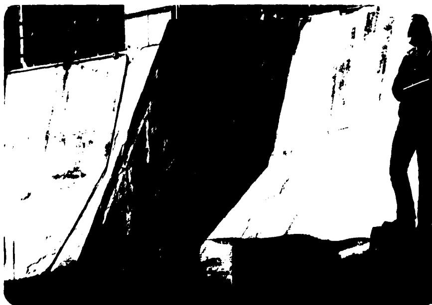
PHOTO C-10: Downstream face of gravity section. Note cracking and efflorescence of concrete.
