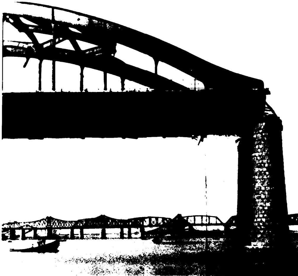
Bridge-busting activities on the Han River
