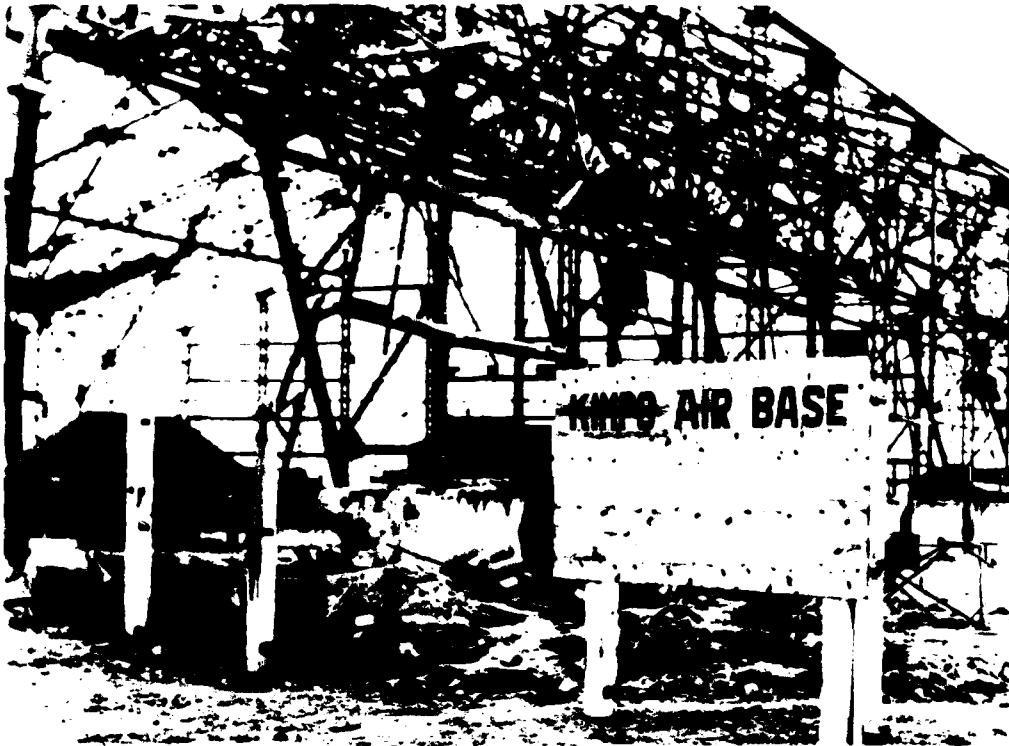
Destroyed hangar and maintenance shop at Kimpo AB
