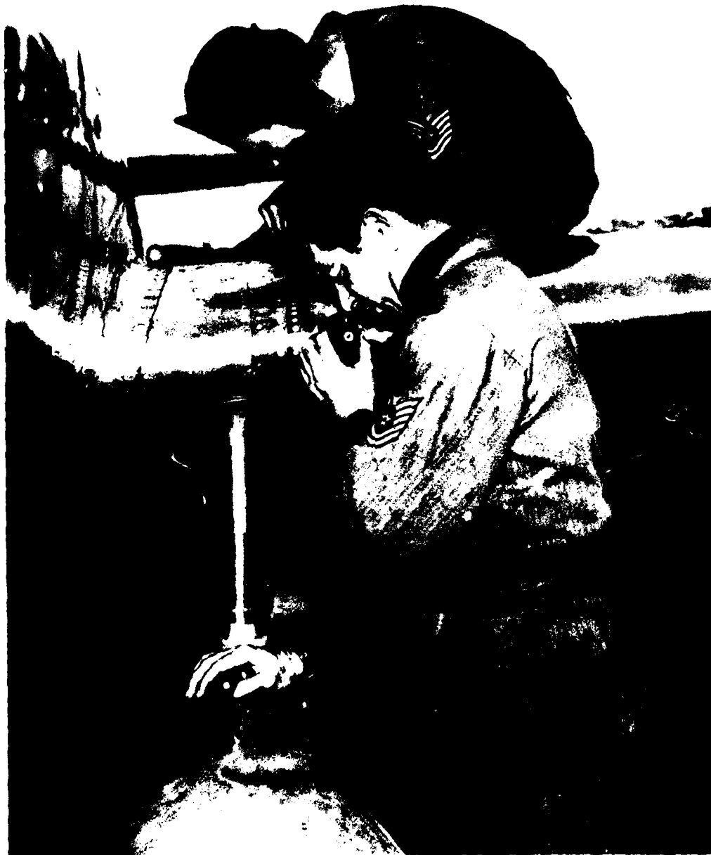
Crewmen boresight the wing gun of an F-84.
