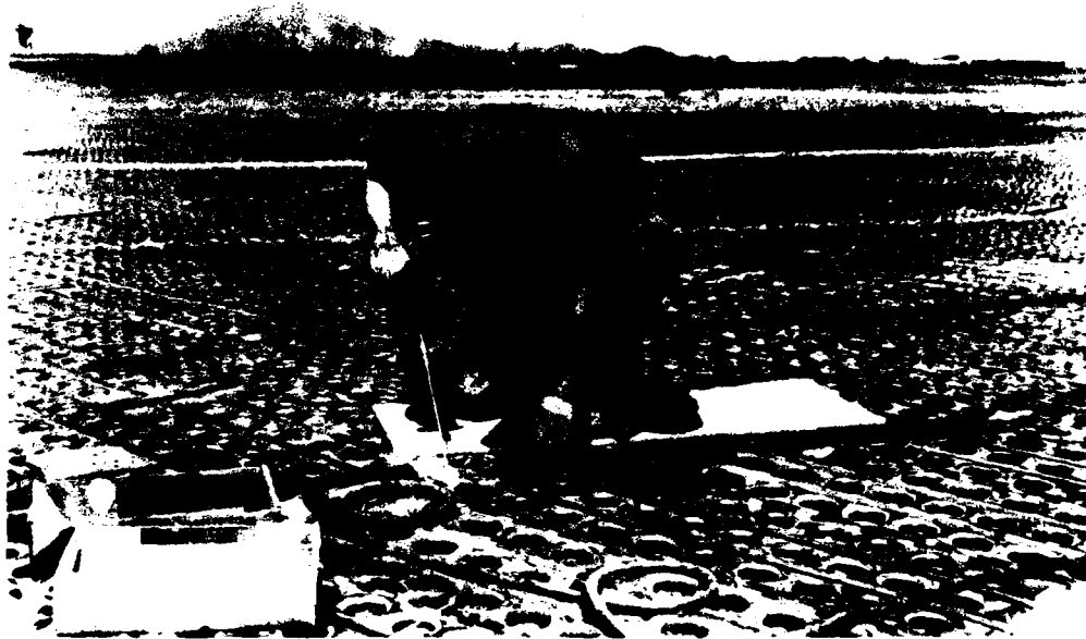
Welding torches were used to repair pierced steel planking
