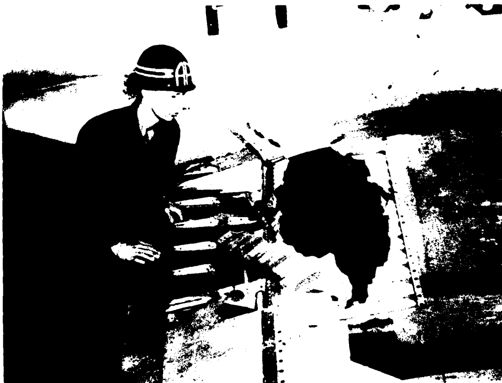
Despite a ruptured fuel tank and wing laceration caused by enemy .50-caliber and 37-mm fire, this RF-80 returned safely to base.
