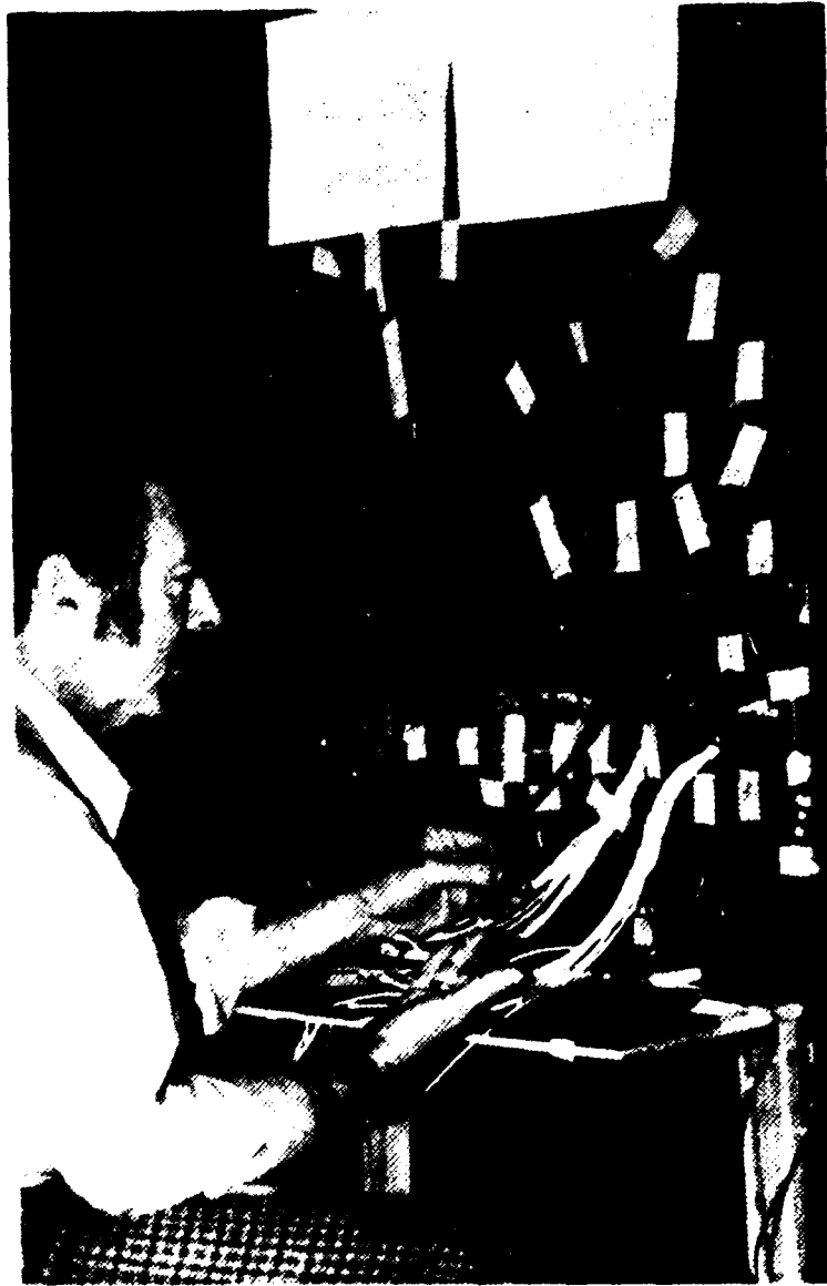
Figure 3 Installing transducers in the oscillating airfoil
