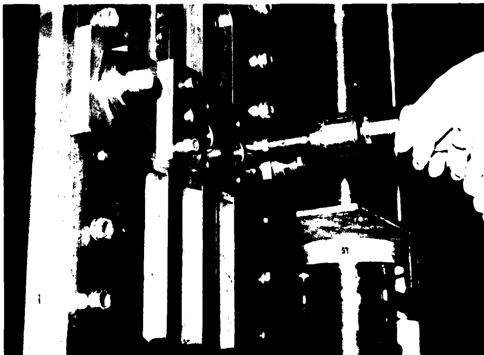
FIGURE 5. HOLE SAW OPERATION TO REMOVE A CRACKED DETAIL
