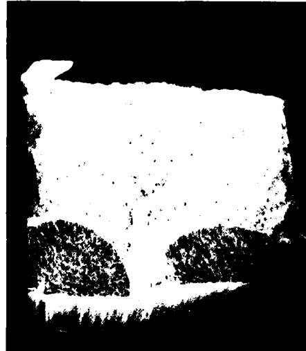
FRACTURE SURFACE - SPLIT FROM CRACKED DETAIL
