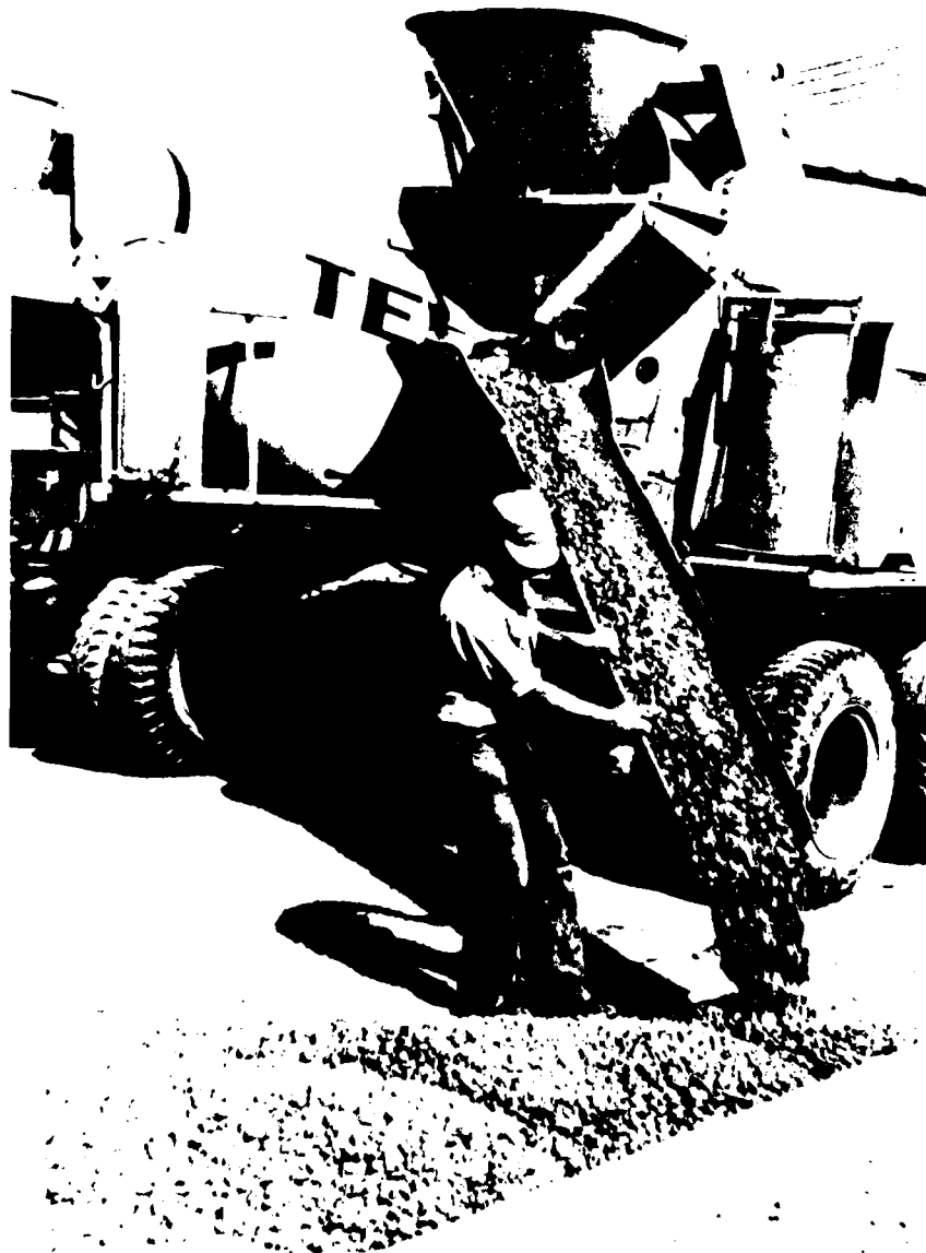
Figure 21. Concrete delivered by revolving-drum truck (photo courtesy of Los Angeles Harbor Department).
