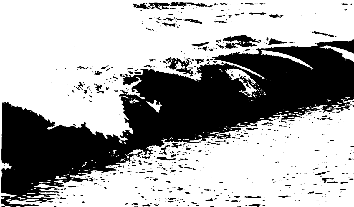
Figure 86. Concrete-filled bags of synthetic fiber used for shore protection (photo courtesy of Fabricast).
