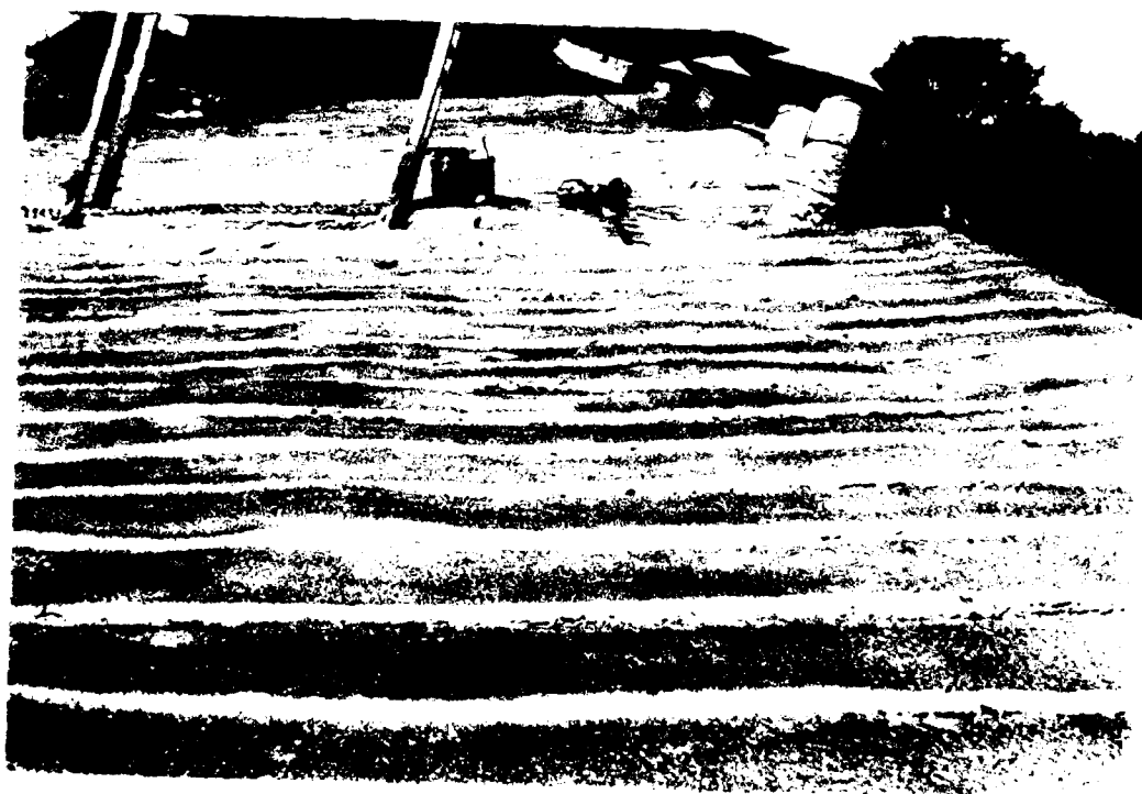
Figure 11. Cracking of silicone coating of System 2 along base of rth. Spraying foam and coating in two directions ("cross hatched") rather than in only one direction would have eliminated the problem.
