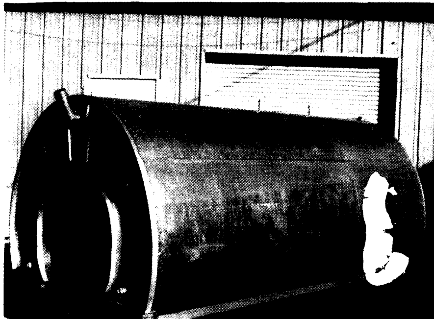
(A) Access Panels Installed
