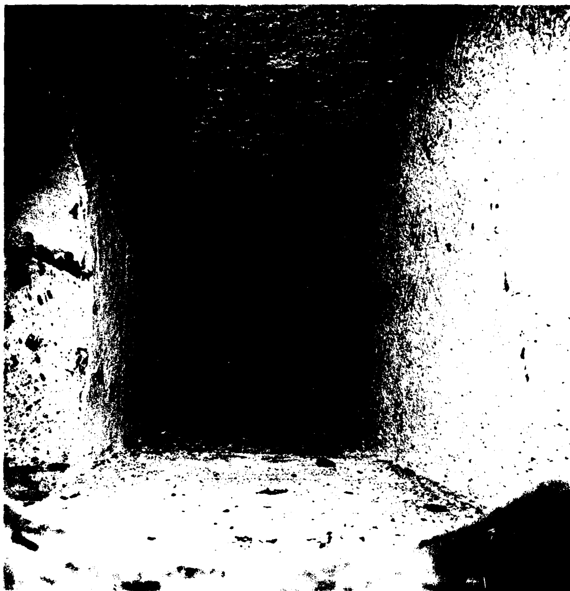
Figure 63. The Cooling Chamber Horizontal Section, with Cured Refractory
