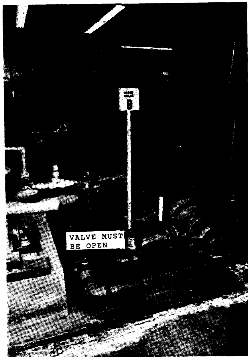
Figure 18, Cooling Water Inlet Valve
