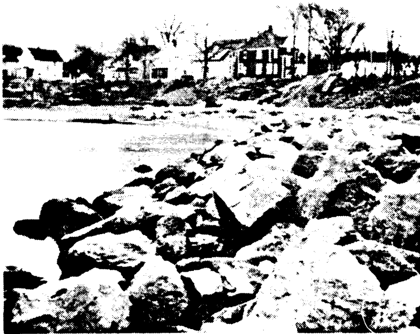
Shoreline at Spending Beach Revetment Spring 1978
