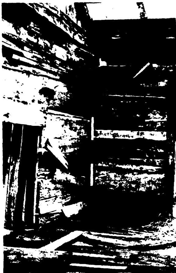
Figure 106. Interior of east corner of the Jim Gilliam dwelling. Note the enclosed fireplace opening at left, the auger hole and notches for the loft floor and the generally dilapidated appearance of the structure.
