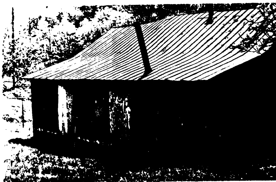
Figure 40. Northern elevation of the McKenzie dwelling showing the board and batten construction of the addition to the log portion of the home. Note rolled metal roofing.
