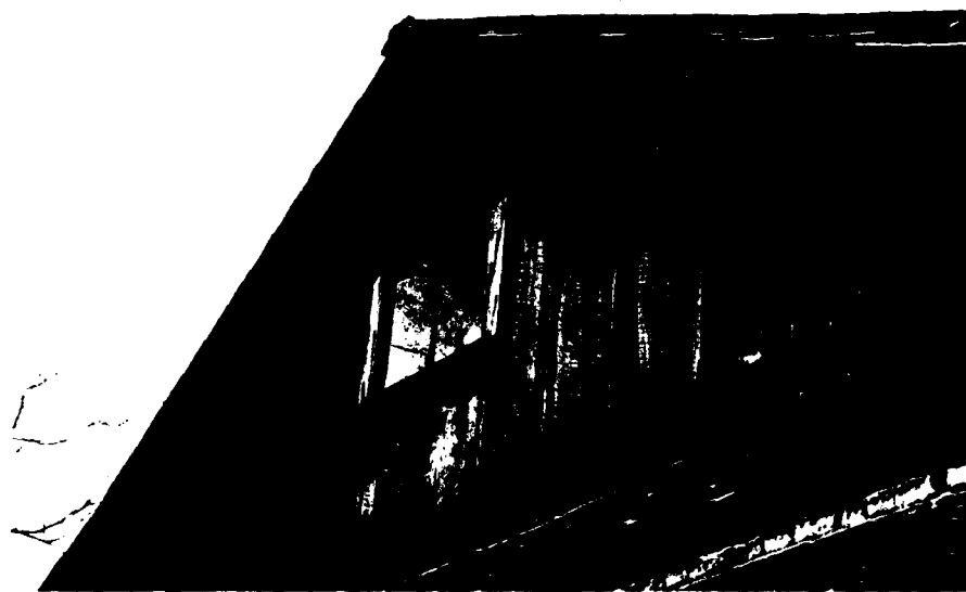
Figure 43. Close-up of plain projecting verge gable on the eastern elevation of the McKenzie dwelling. Contrast vertical application of circular sawed boards on this elevation with their horizontal application on the western elevation. Note, too, that the rolled metal roofing was applied over the pre-existing shake roof on the northern side of the roof while on the southern side, the shake roofing was first removed.
