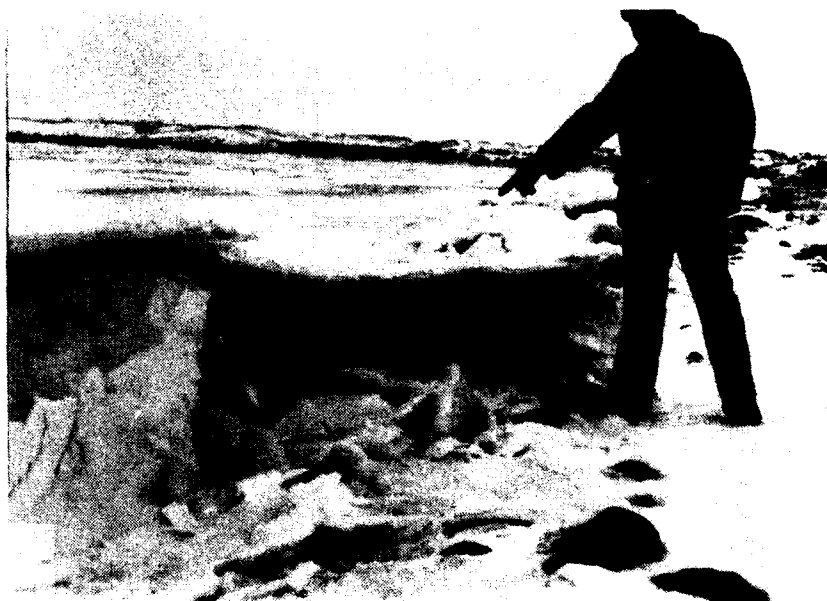
Photo No. 26 - Reservoir ice thrust against riprap along embank- ment upstream berm. Mar 1976.
