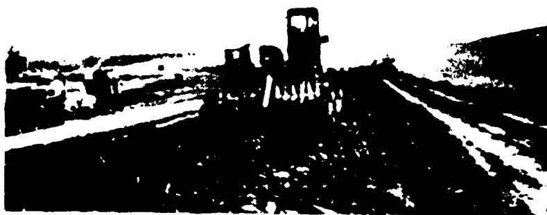
10. Melvern Lake, Construction Photo, Neg. No. 694-R1-10 (Self-propelled tamping roller on embankment fill)
