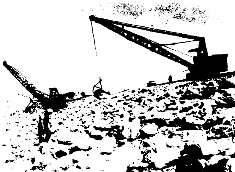
13. Melvern Lake, Construction Photo Neg. No. 88982 (Placement of slope protection on the upstream embankment)
