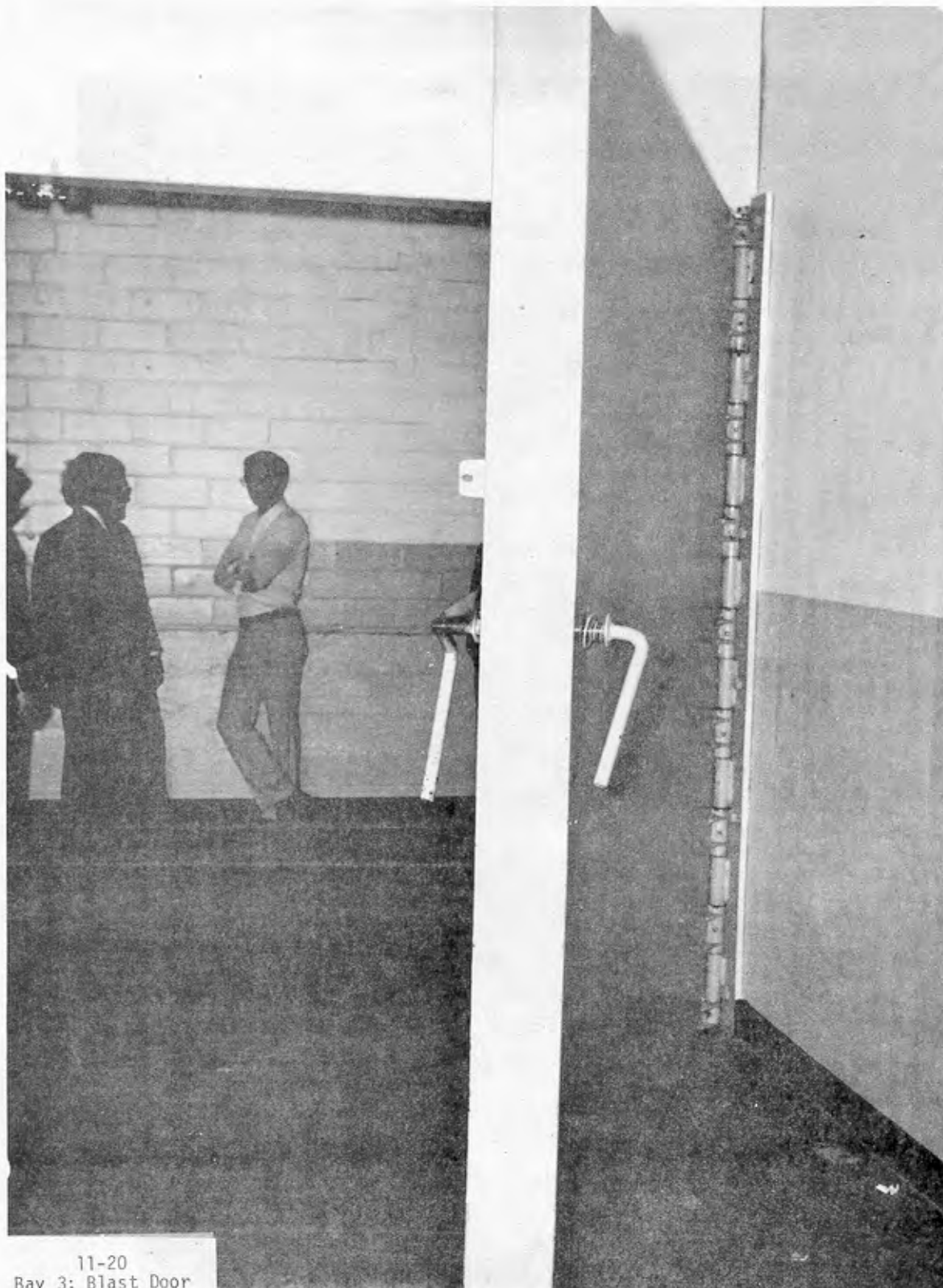
Figure 4.60 Blast Door In Bay 3, Building 11-20
