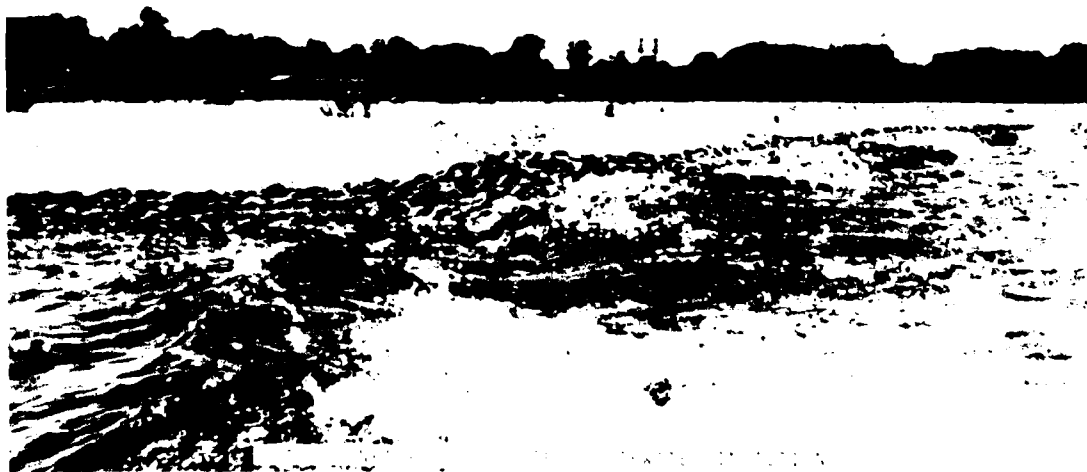
Figure 99. Goodyear scrap-tire floating breakwater concept in operation at Dunkirk Harbor, New York (1976 photo by Goodyear Tire and Rubber Company).
