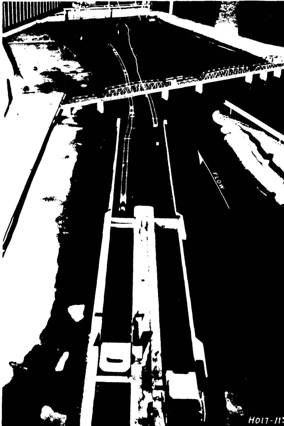
Photo 6. Discharge 246,000 cfs (lower approach). Paths of downbound tow leaving the proposed new 1200-ft lock and upbound tow approaching the existing 1200-ft lock
