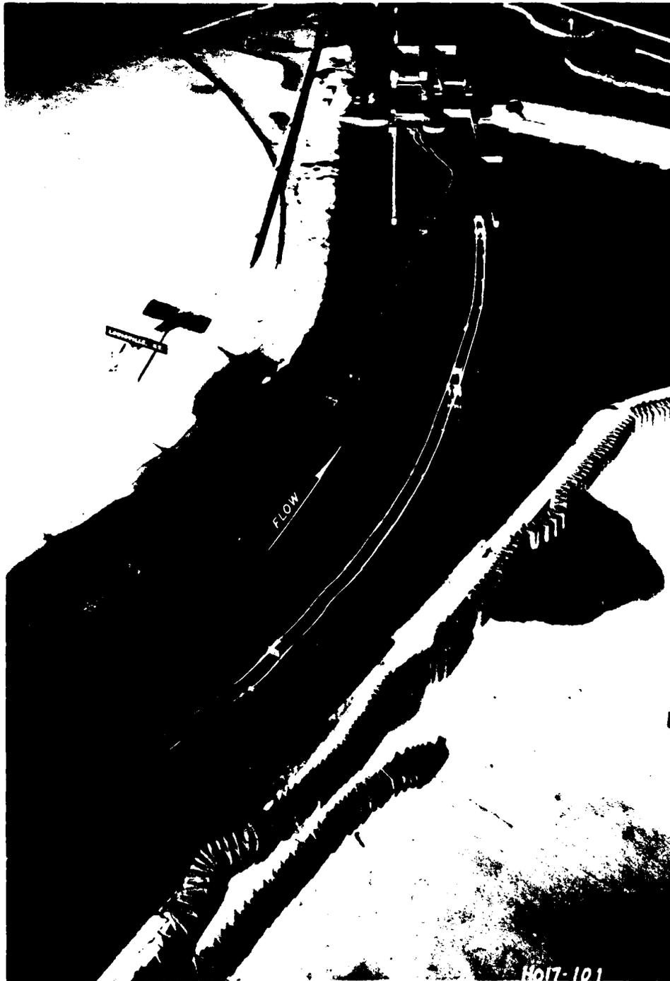
Photo 5. Paths of downbound tow approaching the existing 1200-ft lock and upbound tow leaving the proposed new 1200-ft lock. Note maneuvering required for the upbound tow to turn toward the landside of the canal with slack water in the canal
