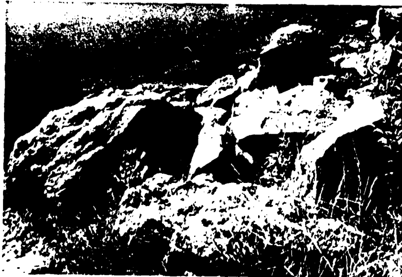
Photo No. 3: RIPRAP ON UPSTREAM FACE
