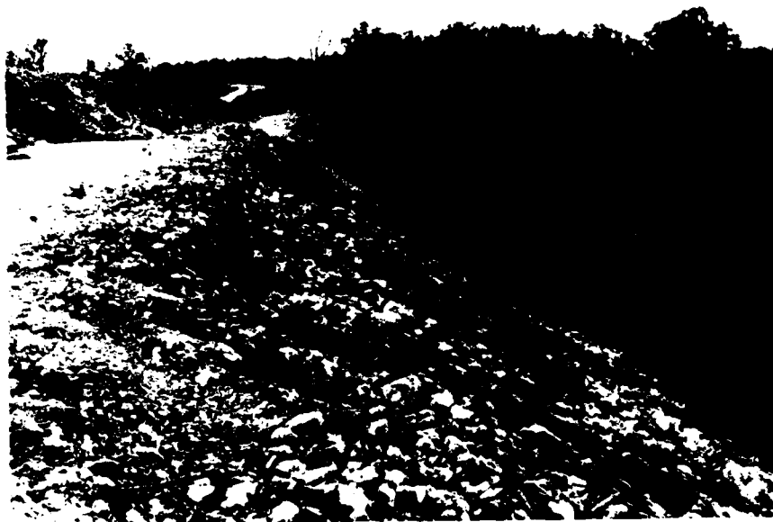
9. Shallow slope failure on lowest tier of downstream face of dam. Looking north.
