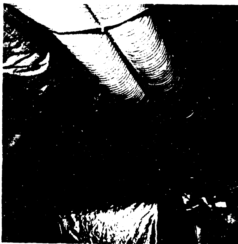
FIG. 16. OVERHEAD 150mm DUCTING
