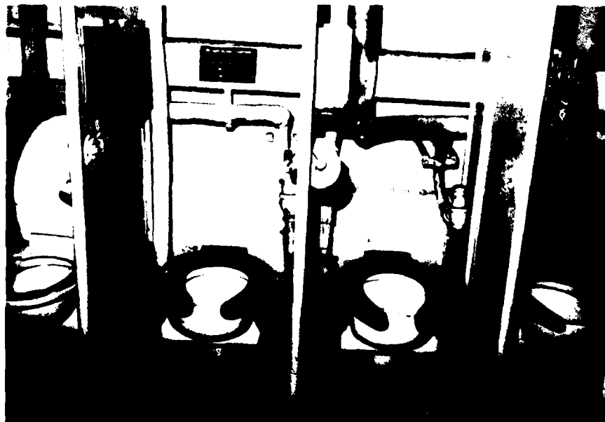
Figure 35. Open Stall Water Closets, Women's Area, USS LEXINGTON (AVT-16)
