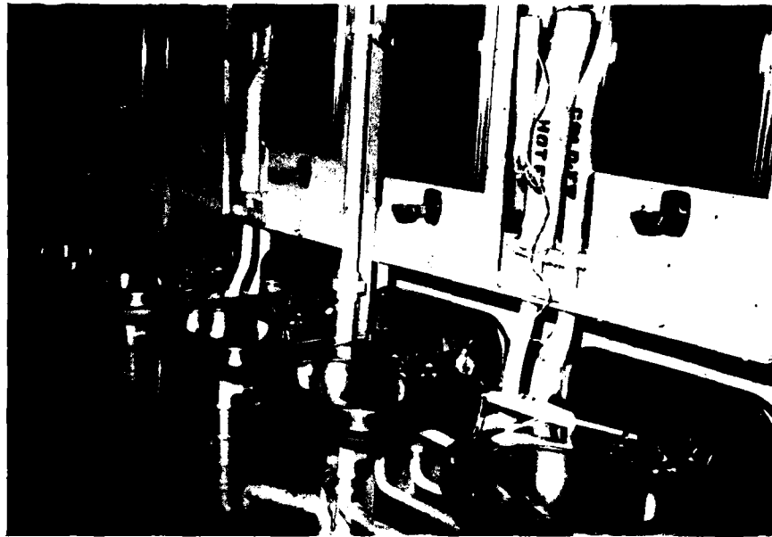
Figure 34. Typical Shipboard Lavatories, USS LEXINGTON (AVT-16)
