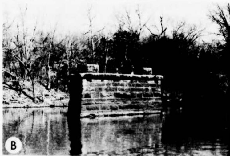
Figure 23 A,B. Site PS-238. A pair of railroad bridge piers built of sandstone are located a little over 3/4 km south of the Adamson bridge on Gaines Creek. These are probably of the 1907 period but possibly earlier.
