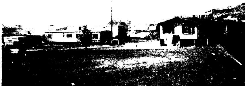
FIGURE 7. TRAILER COURT IN BRIDGEPORT BAR, WASHINGTON.
