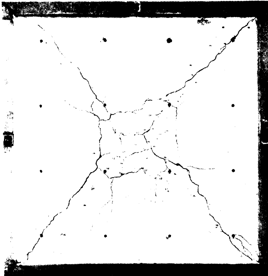
Fig. 50 Underside of a Square Slab G5, Supported on Four Encased Steel Beams, After Collapsing Under 16-Point Loading. The beams were sufficiently strong to prevent the composite beam-and-slab mode of collapse. - Wood (from Ref. 4)
