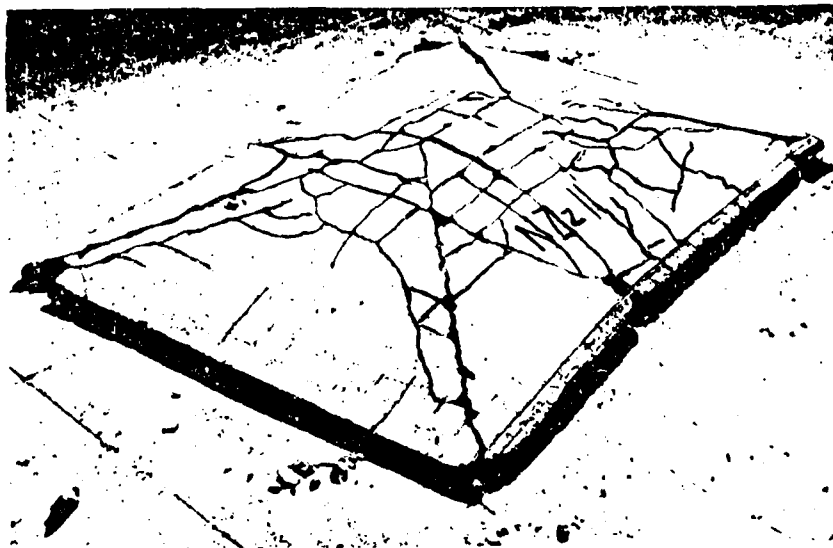
Fig. 62 Permanent Deflection of a Slab Due to Membrane Action and Bending - Sawczuk and Winnicki (from Ref. 18)
