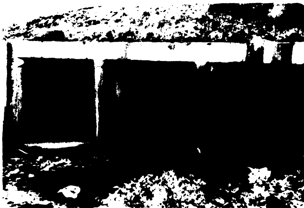
PHOTO # 10 TRIPLE BARREL BOX CULVERT THRU I-77 EMBANKMENT
